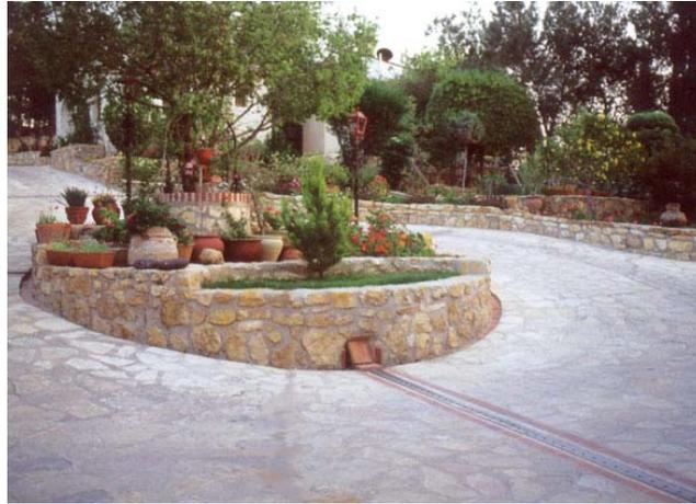
**Fig. 2.2: Hardscaped surfaces serve to collect and channel rainwater as part of a water harvesting system.**
