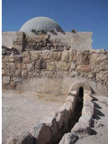
**Fig. 3.3: A historical example of water harvesting at the Amman Citadel. Water collected from the roof is directed through channels towards water storage areas.**
